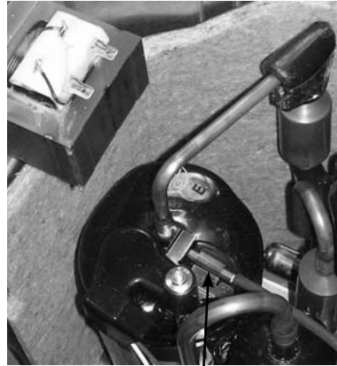
Discharge temperature thermistor
